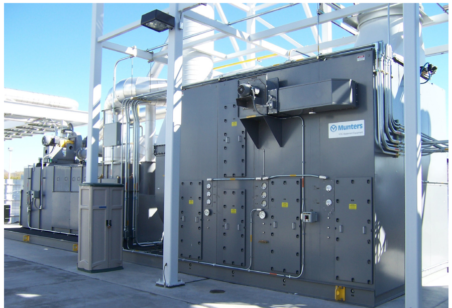
Munters Installation at ST Microelectronics, Phoenix, AZ
